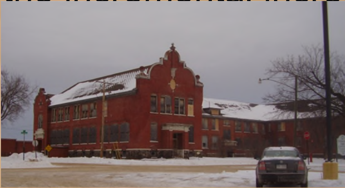
Central School Iron River
